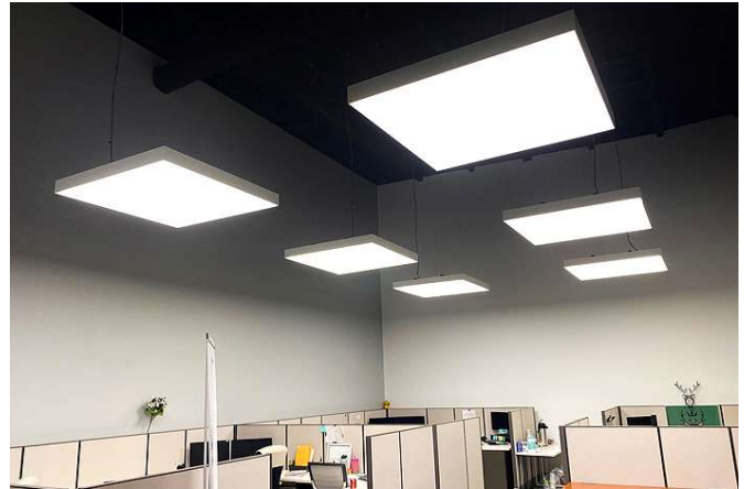
A new generation of acoustic lighting fixtures is now available that deliver a clean design, provide high quality illumination, and provide a significant contribution to the overall acoustic comfort in open concept spaces with exposed ceilings
