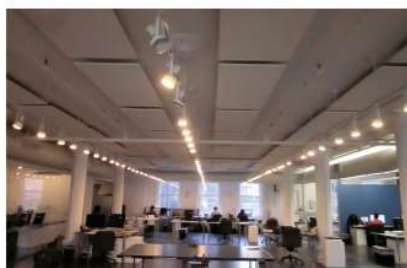
Dozens of bright point sources are used to provide general illumination to make room for acoustic panels
